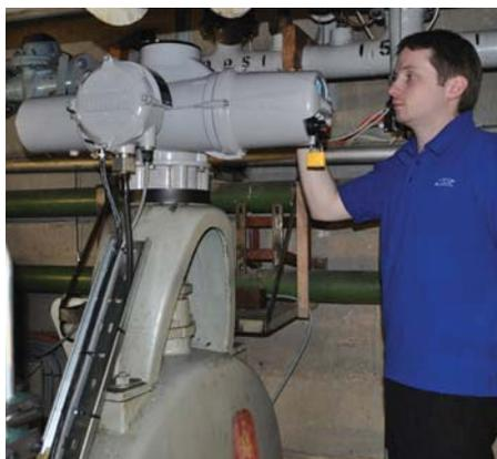
new IQ3M actuators that are specifically designed for modulating duties. Because there is a constant demand to use the wind tunnel, the retrofit operations can be completed in the brief periods available between test programmes. The first two actuators were removed and the replacement IQ3M actuators installed and commissioned in two days, half the allocated time allowed before the wind tunnel was due to re-start operations.
